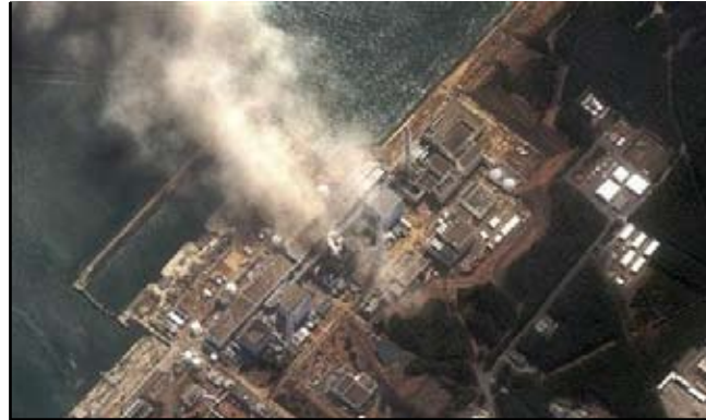
The containment at the damaged nuclear power plant releases a dangerous plume.
